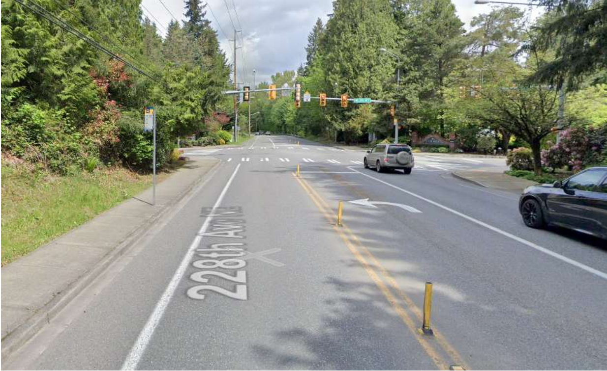
FIGURE 7: NARROW SIDEWALK AT THE BUS STOP AT 228 TH AVE NE/NE 25 TH WAY
