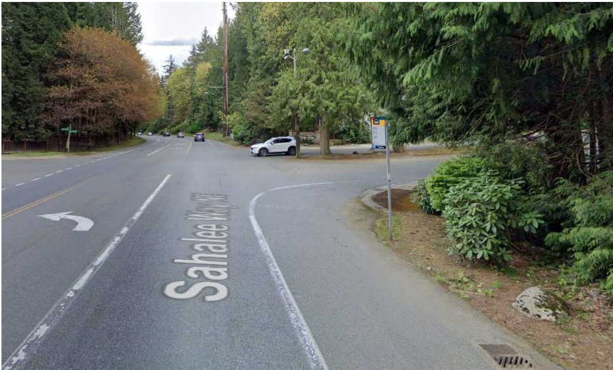
FIGURE 6: NO SIDEWALK AT THE BUS STOP AT SAHALEE WAY AND NE 28 TH PL/223 RD AVE NE
